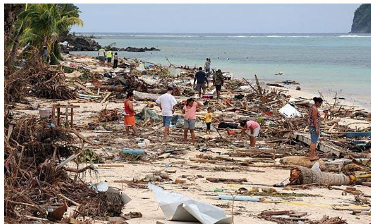
Figure 11A: Destroyed structures in the aftermath of the tsunami (Source: divinationpower.com)
