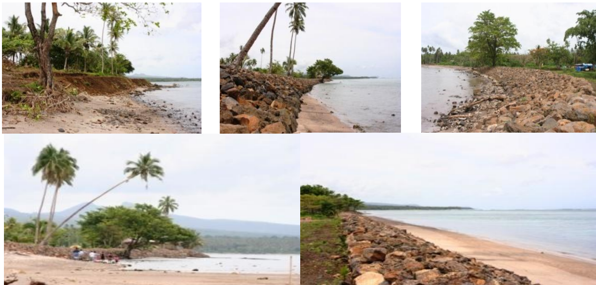
Figure 14: Multiplication of seawalls, affecting aesthetics of Samoan coast (Source: By author).
