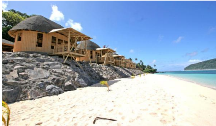
Figure 11B: Beach fale accommodation rebuilt at the same place (Source: Samoan Observer, 16/08/2010).
