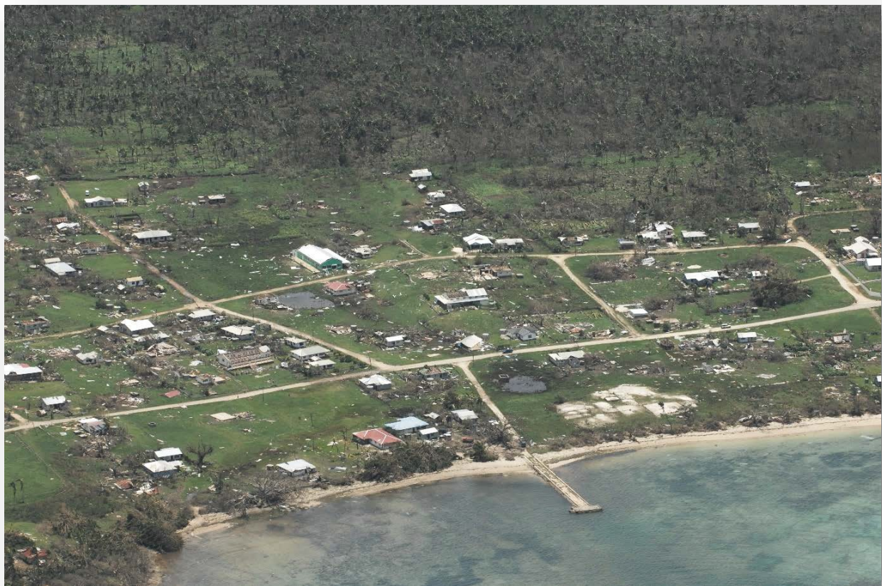
Figure 4.2 Aerial view of damage to Foa and Foa wharf. Source: Tonga NEMO, 2014.
