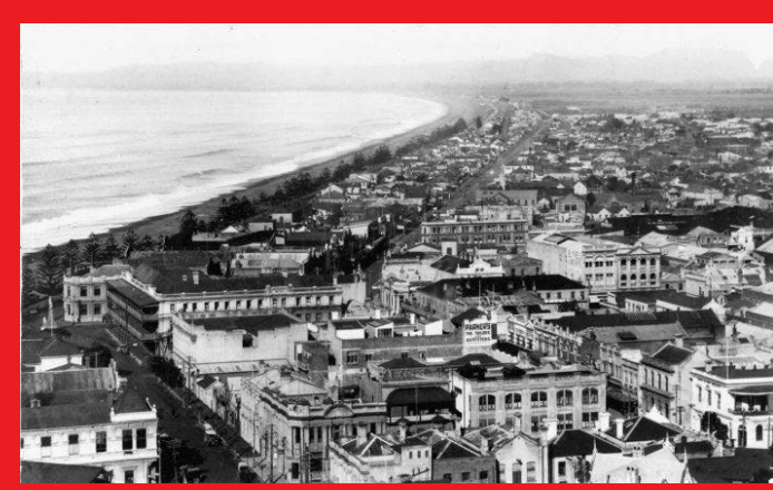
Napier Central Business District in 1929 (P.C. Sorrell / A. Turnbull Library)
