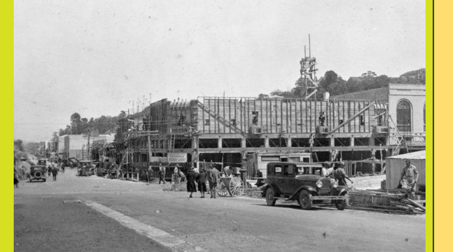
Rebuilding in central Napier including resistant framing and splaying of the corner (Anonymous / A. Turnbull Library)
