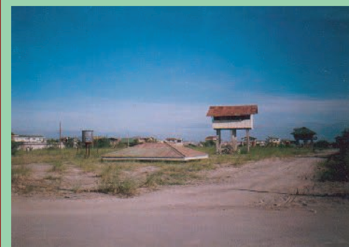
Fig. 3. Houses raised on concrete posts in Cabambangan, Bacolor, in December 1997 (JC Gaillard)
