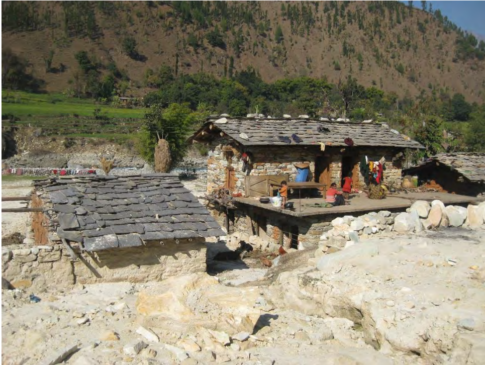
Picture 45: Rocks piled up to limit the landslide impact, Bangabagar
