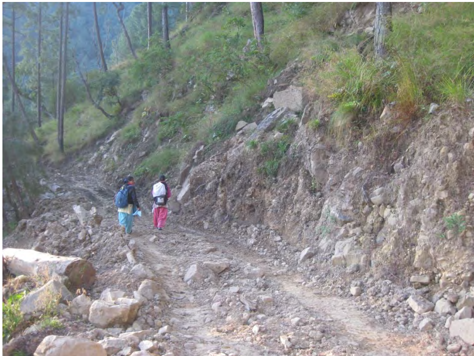
Picture 23: Recently built feeder road to Shivanagar, Nigali
