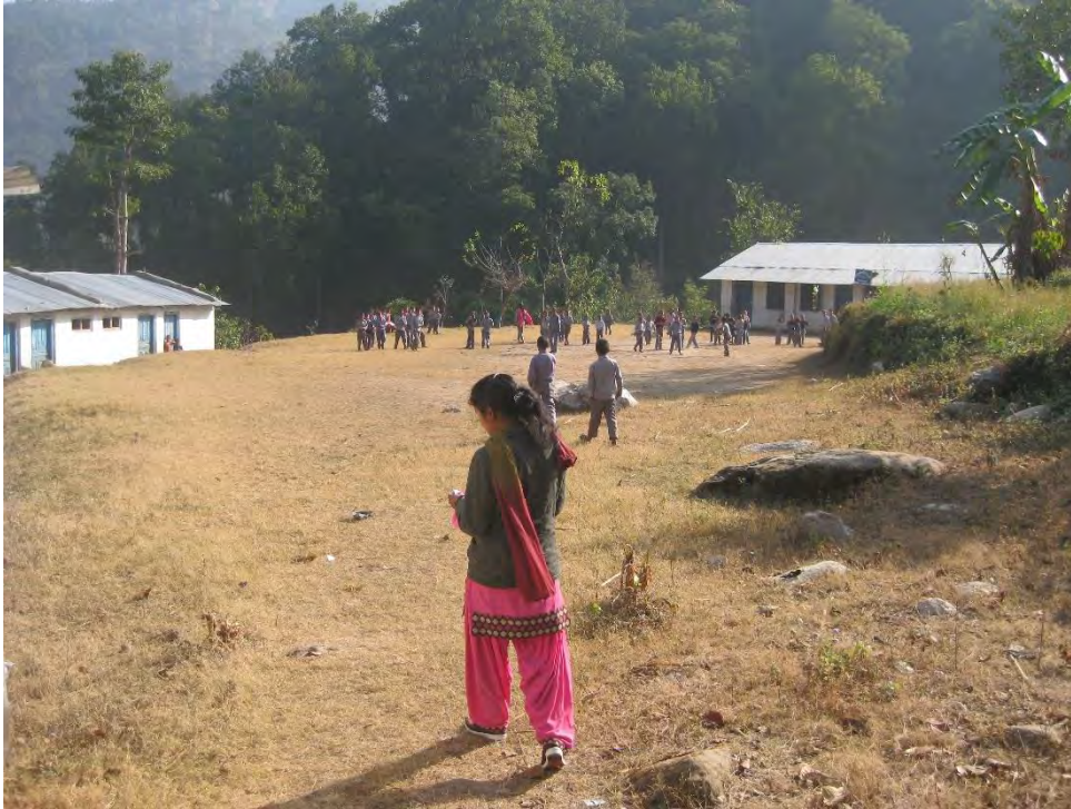
Picture 61: Reconstructed school (now moved to safer land)
