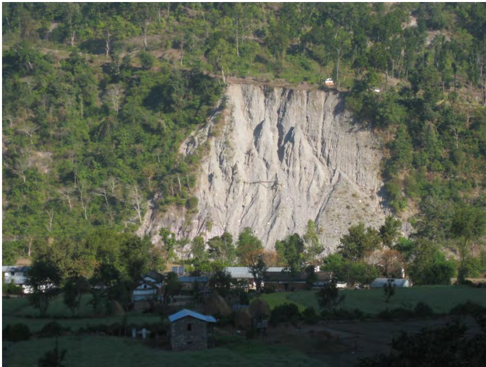
Picture 35: Erosion in Shivanagar, Nigali
