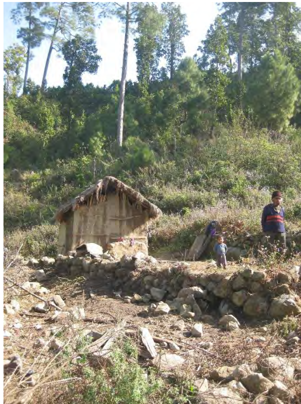
Picture 58: Temporarily fixed hut just below the landslide, Patreni
