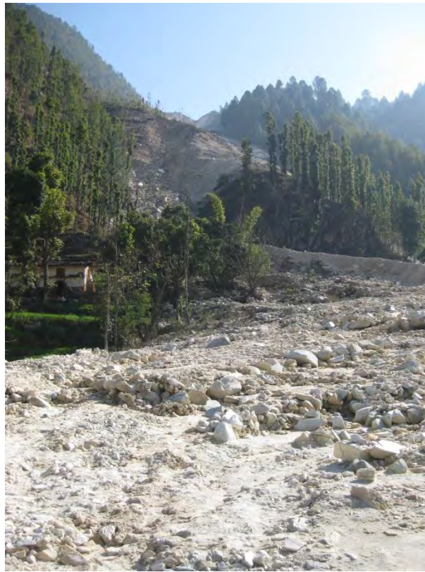
Picture 38: The expanding landslide, Bangabagar
