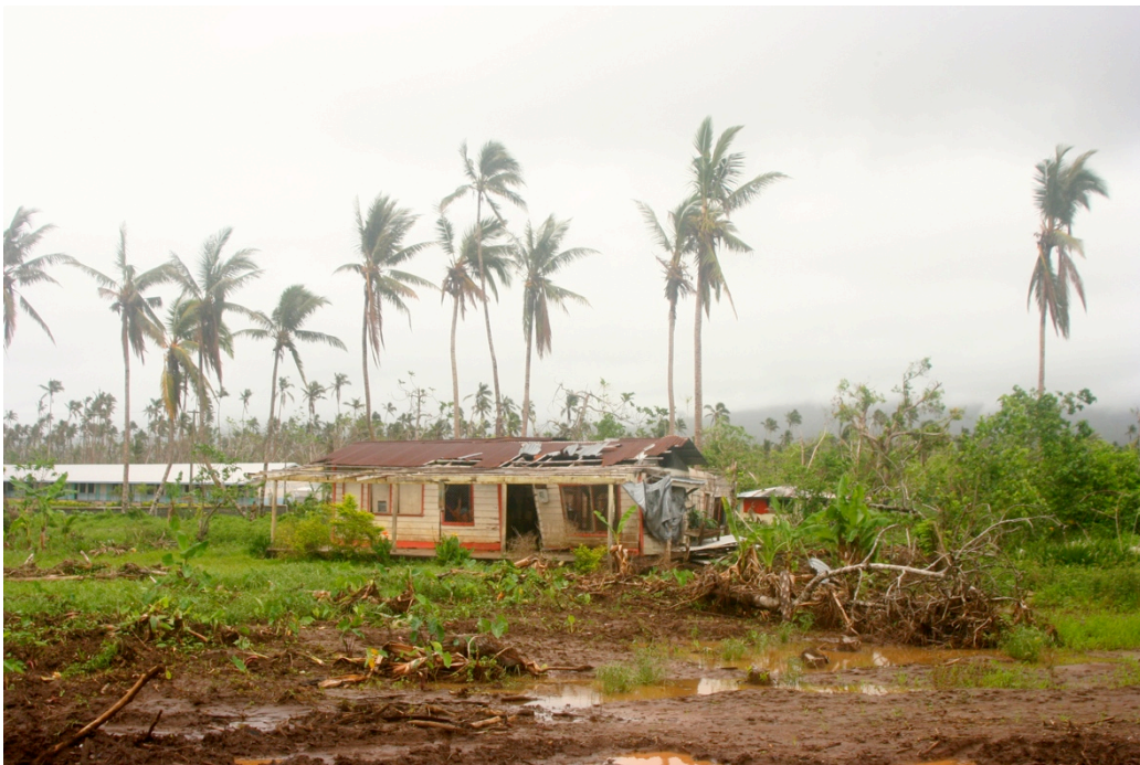
Figure 8.1: Damages from the 2012 cyclone Evan, Tafitoala village, Samoa
