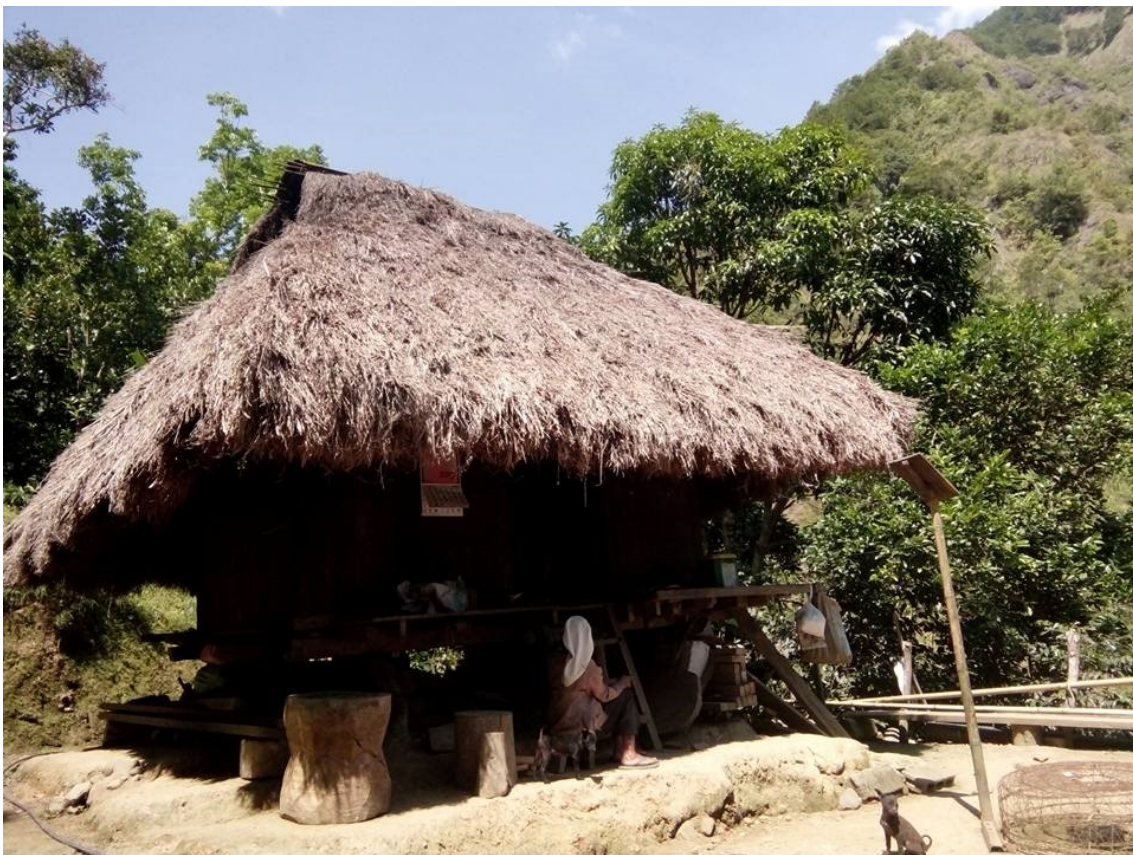
Figure 3.1: The inatep or traditional Kankanaey house that stands on four pillars – Photo by Charleston Pasigon, June 2016 (Photo used with permission).
